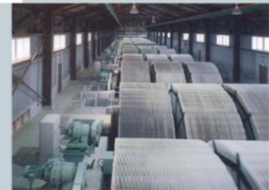
In fig 2- rotating bio-discs are arranged together in STP ( no. of bio-discs also matters)
